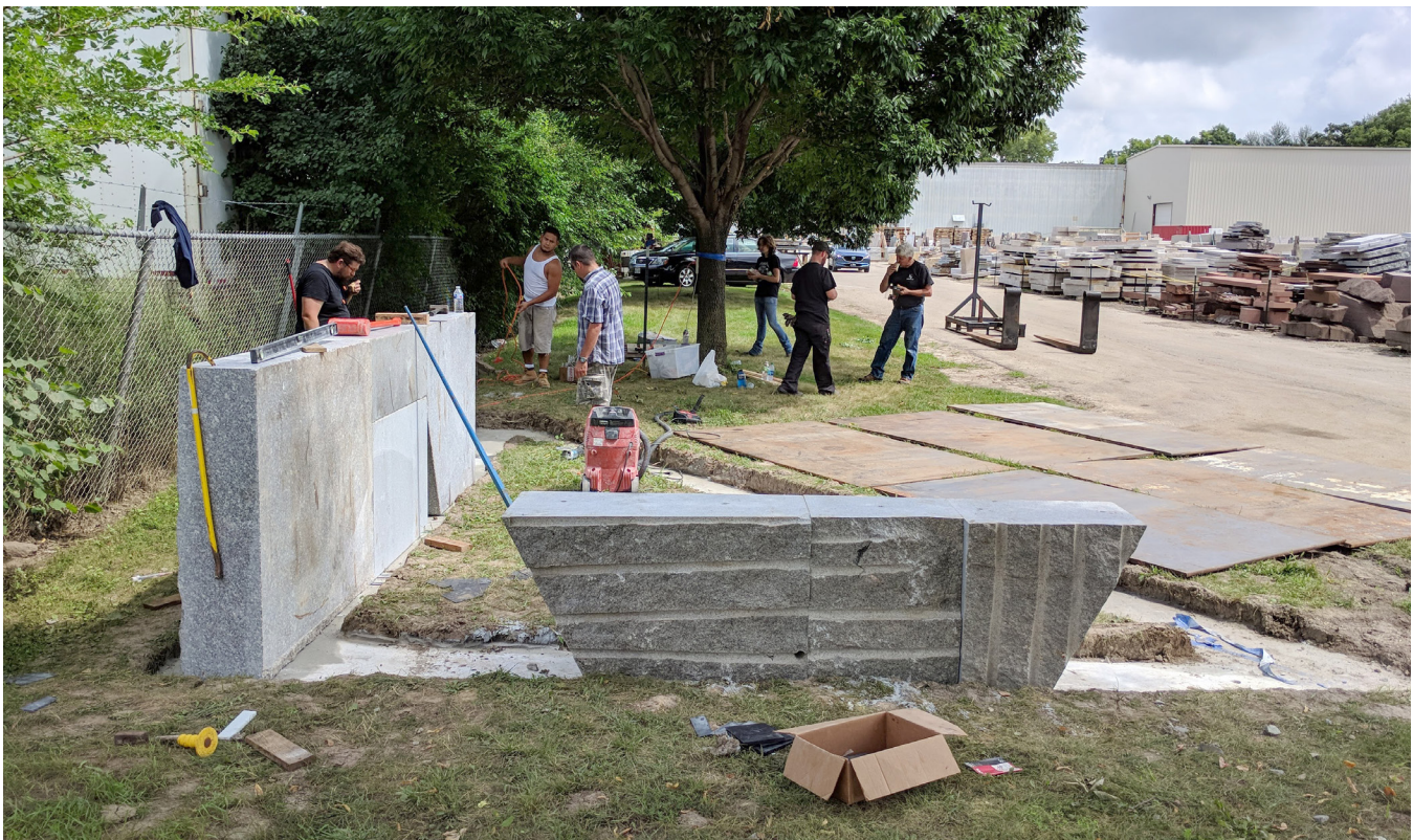
Figure 1. Granite Wall Construction Process. Photo by Author.
