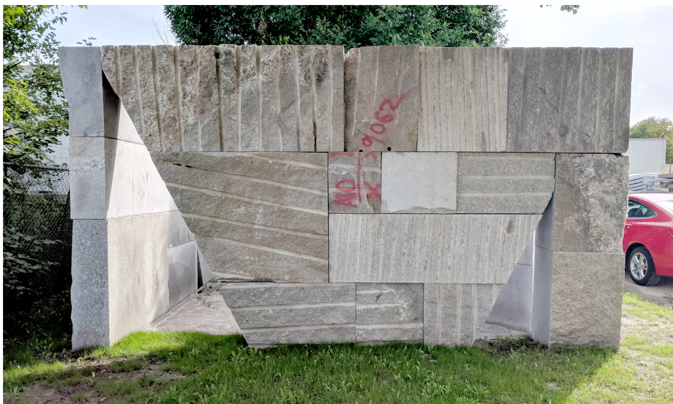
Figure 3. Granite Wall Completed Assembly. Photo by Author.
