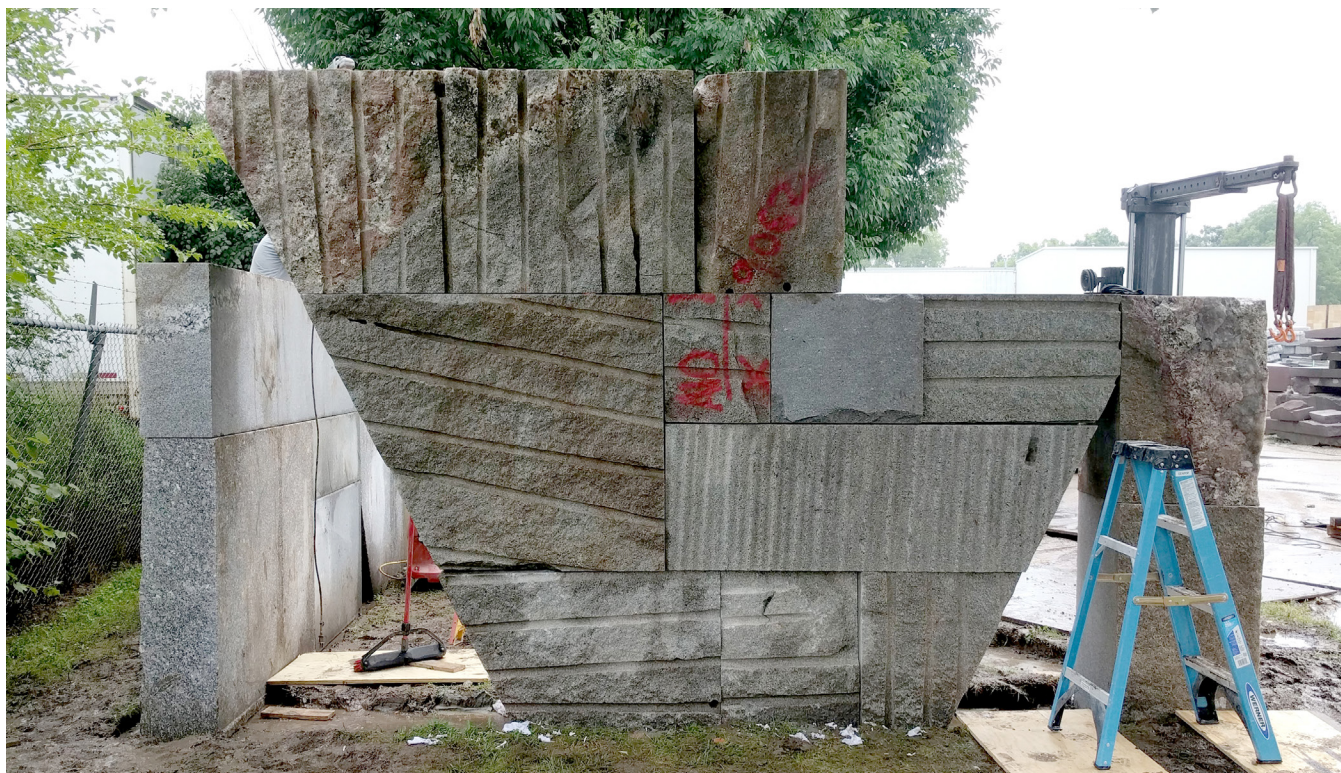
Figure 2. Granite Wall Construction Process. Photo by Author.
